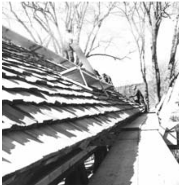
Re roofing the Bradford Bridge
