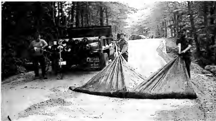
Fairgrounds Road – paving fabric installation
