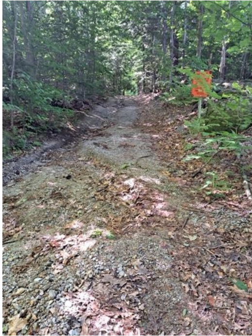
Entrance to Blaisdell Hill Road 2024
