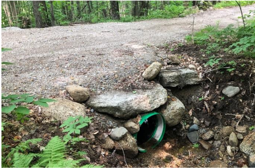
New Culvert on Rowe Mtn Road 2022
