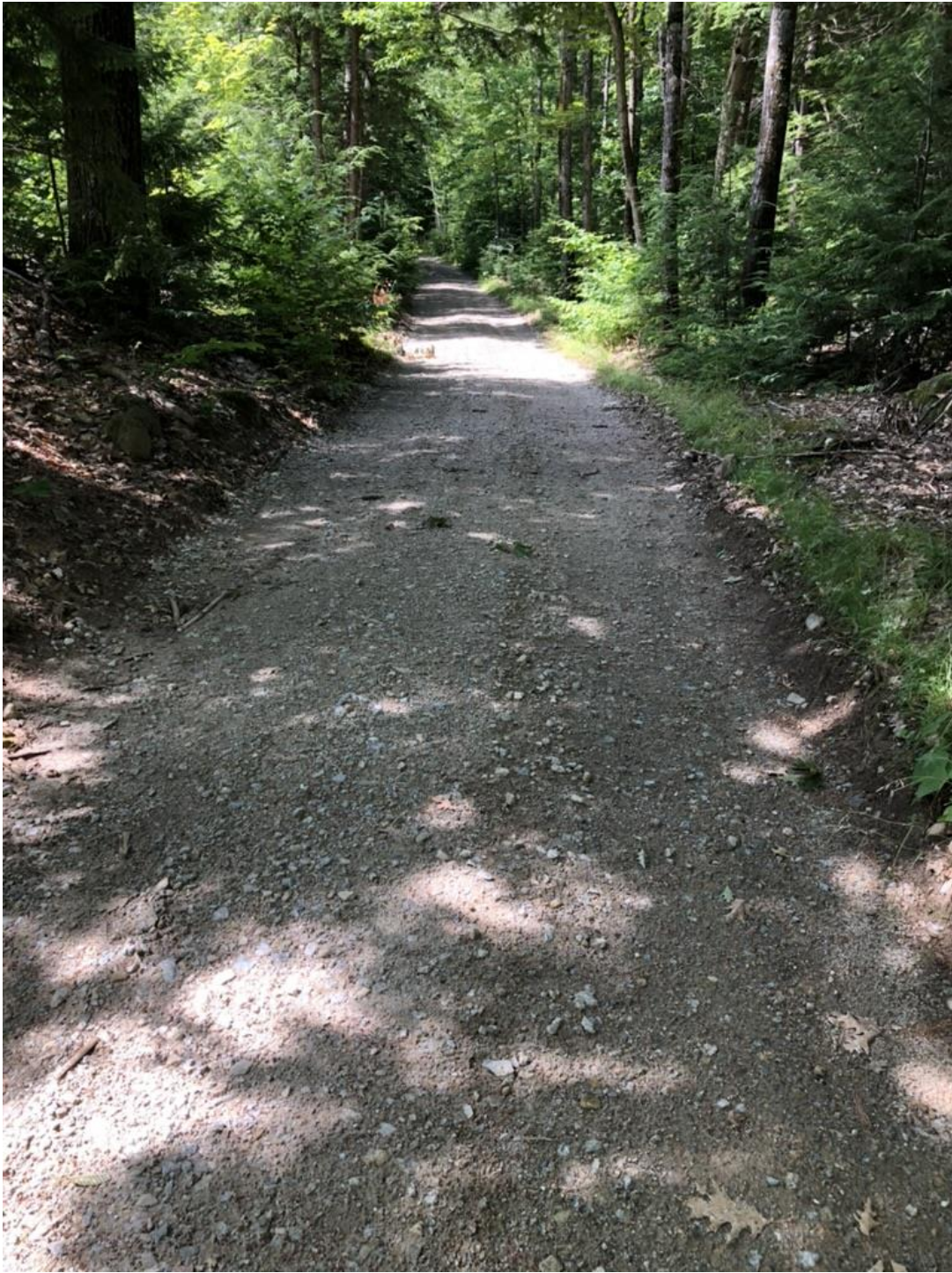
Privately Upgraded Road Surface July 2024
