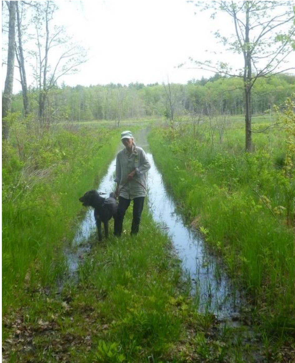
Submerged Section of Alder Plains Road 2022
